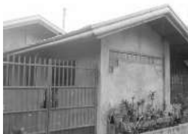
Fig 3. Cement Exterior Wall and G.I. Sheets Roofing
